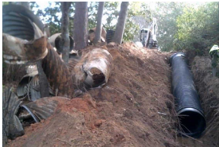
Photo 39: Stormwater line repair
