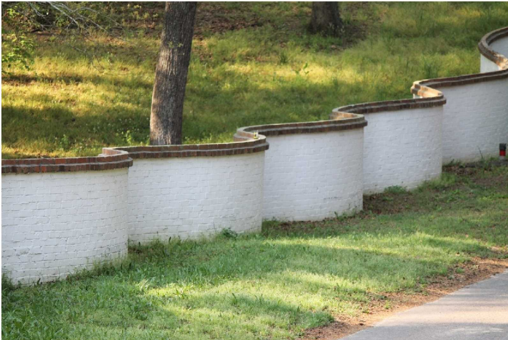
Photo 69: Serpentine wall at Banksia
