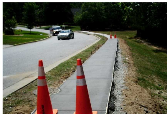
Photo 36: Safety cones mark sidewalk improvements
