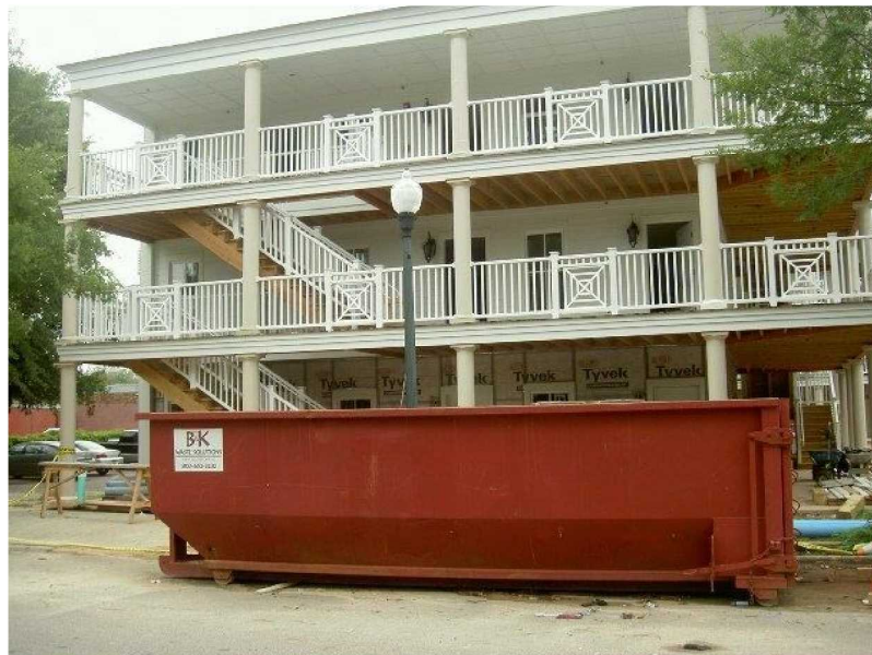
Photo 55: Renovations in progress on the Carriage Park Inn
