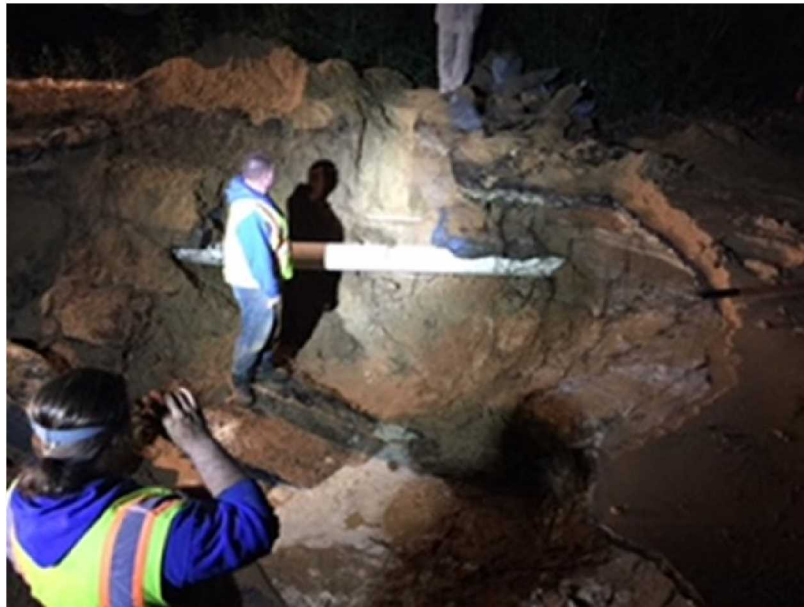
Photo 38: Major repair on a water main
