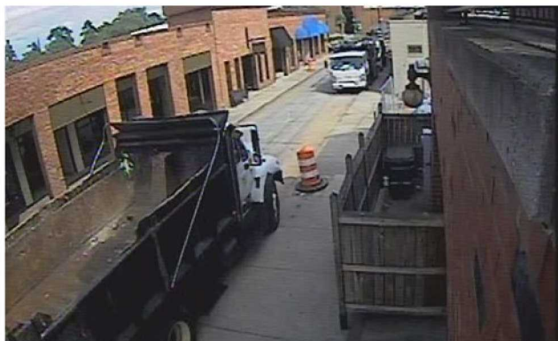
Photo 23: Improvements to the Alley, in progress
