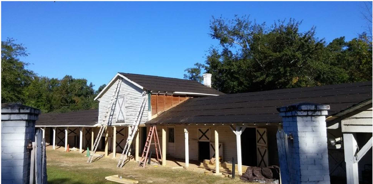
Photo 13: Rye Patch stable renovations in progress
