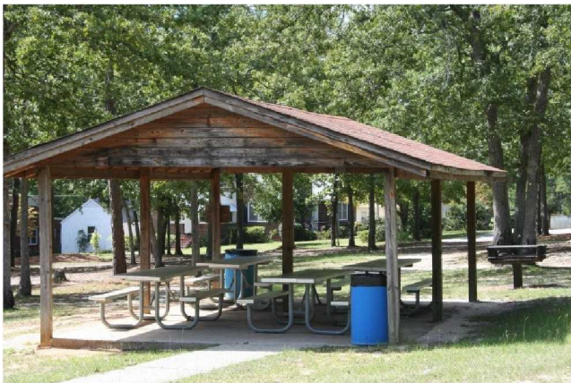
Photo 71: Eustis Park picnic shelter
